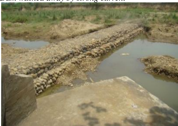
Dam constructed with Sausage wire & boulders
