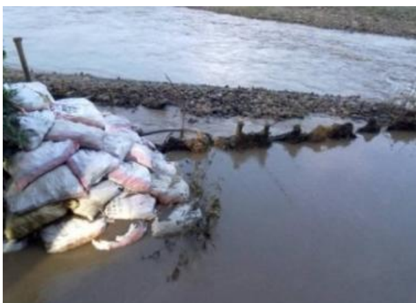
Dam washed away by strong current
